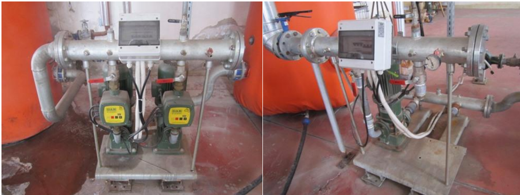
Pompe transfer apa cu tablou electric DAB Activer Driver - 4 bucati
